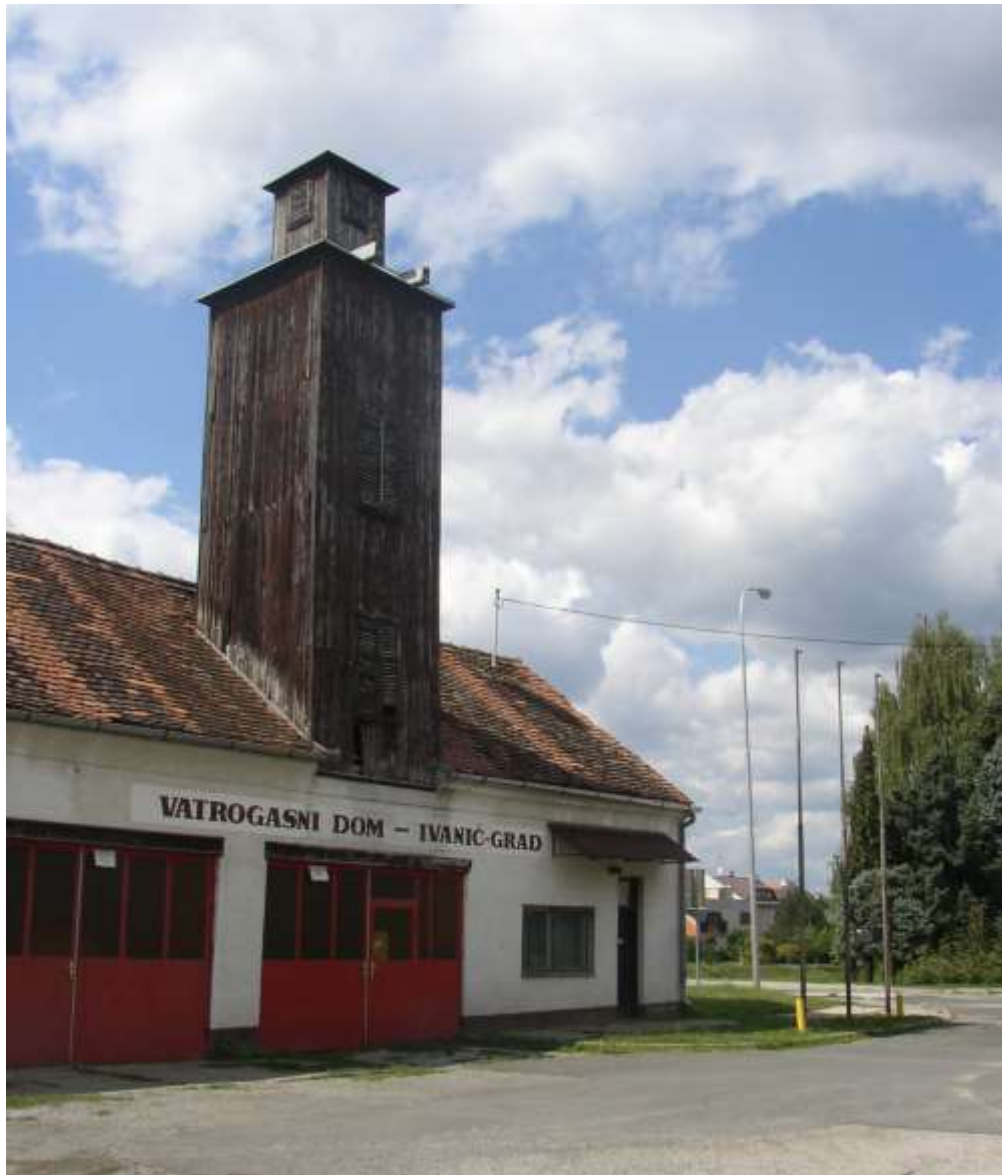
The Ivanić-Grad old Fire station built in late 19th century
