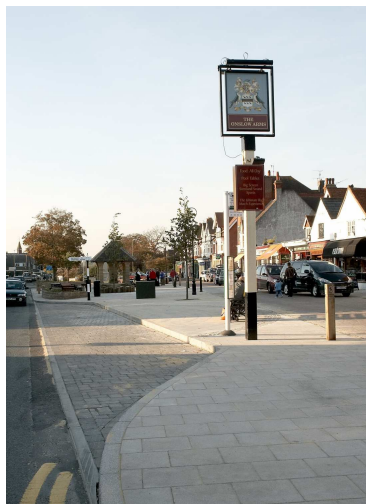
Left: Picture of town centre improvements, Cranleigh
